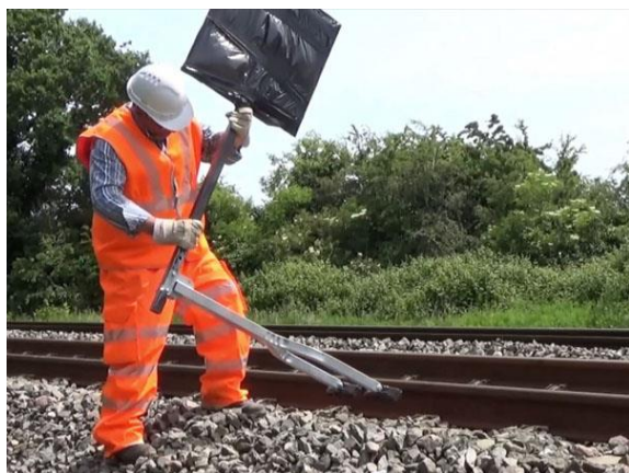
CLOSURE DUE TO RAILWAY WORKS
